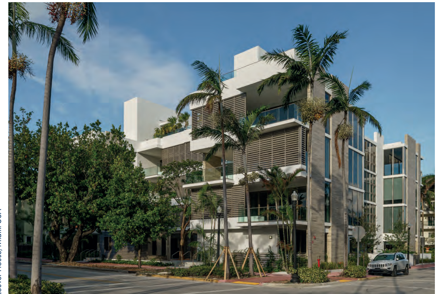
Louver House, Miami USA
