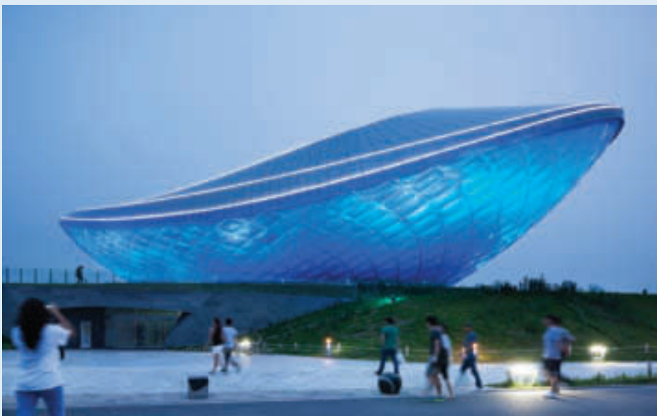
ARC River Cultural Pavilion, Daegu, South Korea
