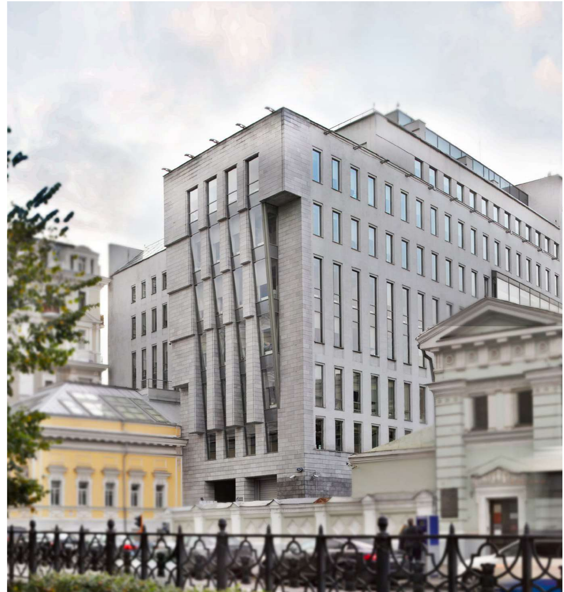
The office building is in historic downtown Moscow—the Boulevard Ring Road. Here, next to Pushkin Square and Tverskaya Street, is where high-end hotels, luxury housing, restaurants, salons and shops are located. The favourable location gives convenient access to all major thoroughfares of the capital, including Sadovoye Ring Road and Leningradsky Prospekt.
