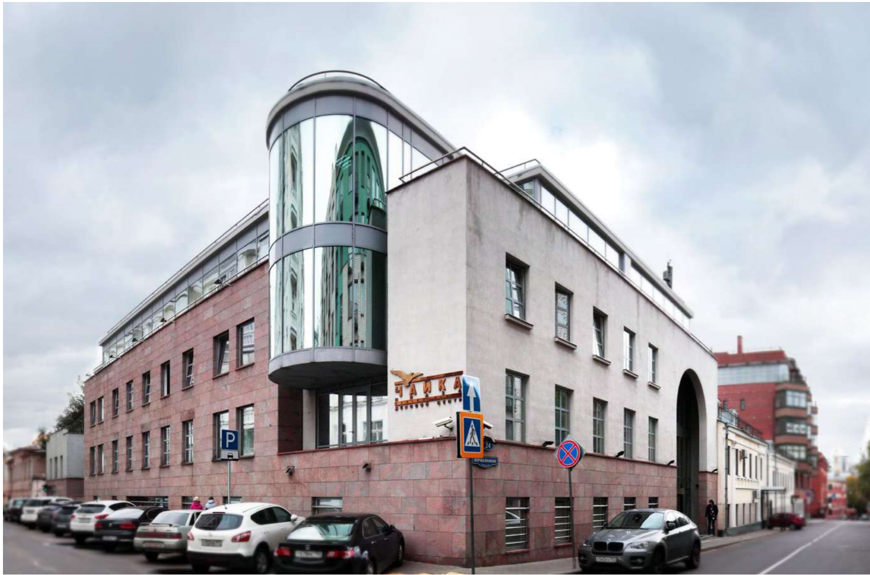
This four-story office block is located in the unique historic district of Ostozhenka, a quiet area in downtown Moscow. In the immediate proximity are the Kremlin, the Cathedral of Christ the Saviour, and a number of business centers and embassies.
